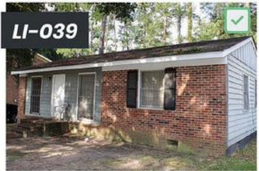
Single Family Residence: Albany, GA
